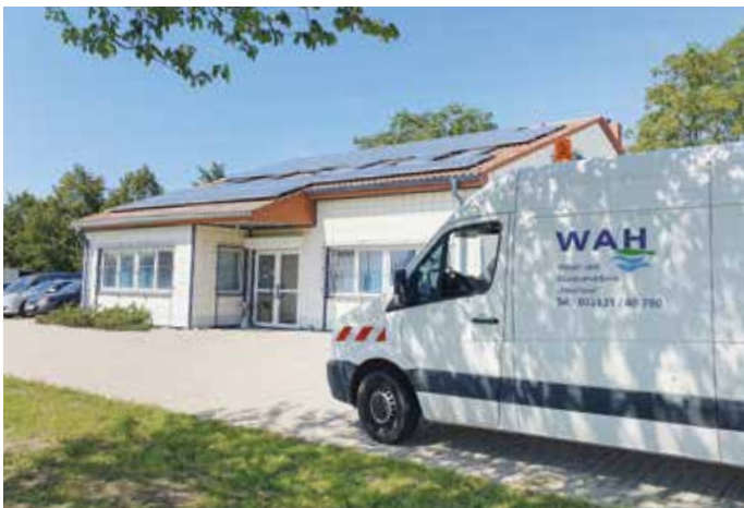
The Roskow wastewater treatment plant is now up to date in terms of energy efficiency and has been able to significantly reduce its energy consumption, CO 2 emissions and costs as a result.
