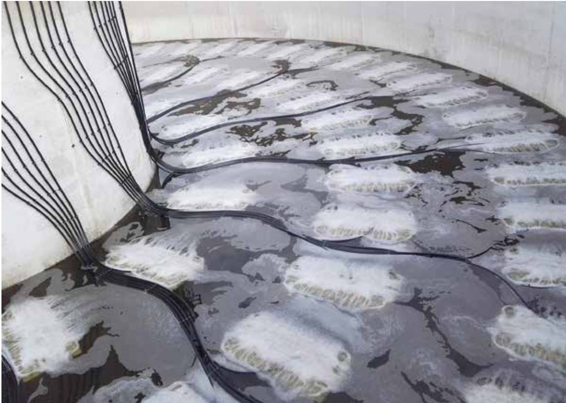
New aerators ensure that the air provided by the AERZEN packages reaches the pool. As a result, the oxygen input is 50 % higher than with the old candle aerators.
